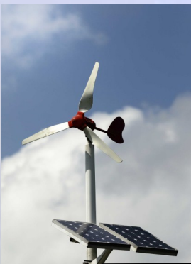
Wind generator with Solar panel, diameter 1.5 m
